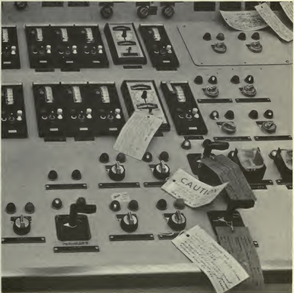
Control panel of TMI-2, showing maintenance tags that operators testified covered one of the closed emergency feedwater valve indicator lights during the first 8 minutes of the accident.
